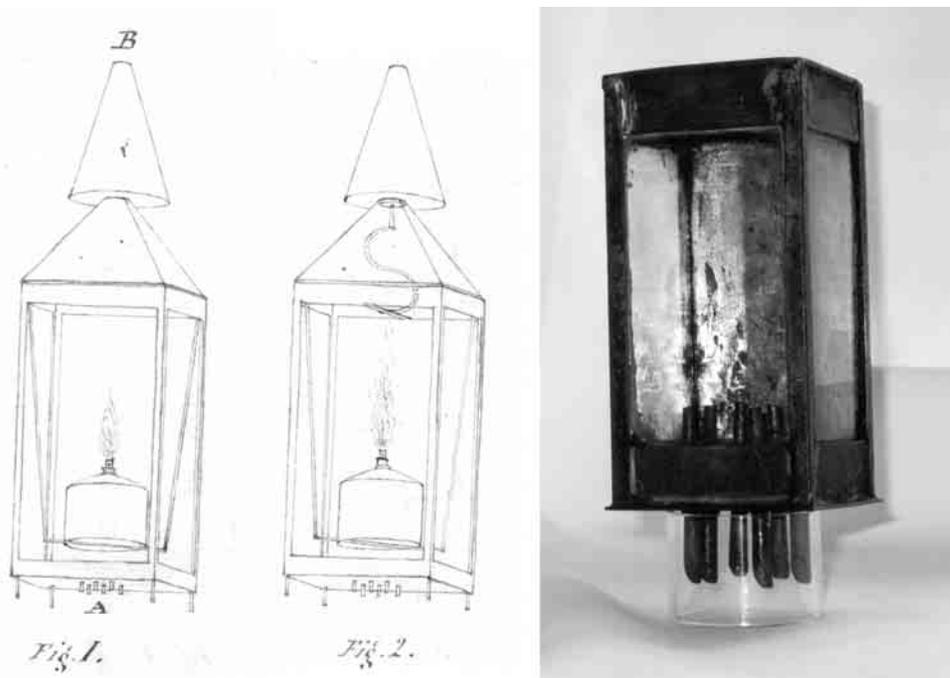
Fig. 12. Davy's lamps with  $1\frac{1}{2}$  inch intakes. (a) the Safe Lamp, (b) the valve lamp (both drawn by Faraday in RI MS HD 11, p. 111) and (c) the bottom half of the lamp in the Collections of the Royal Institution.
