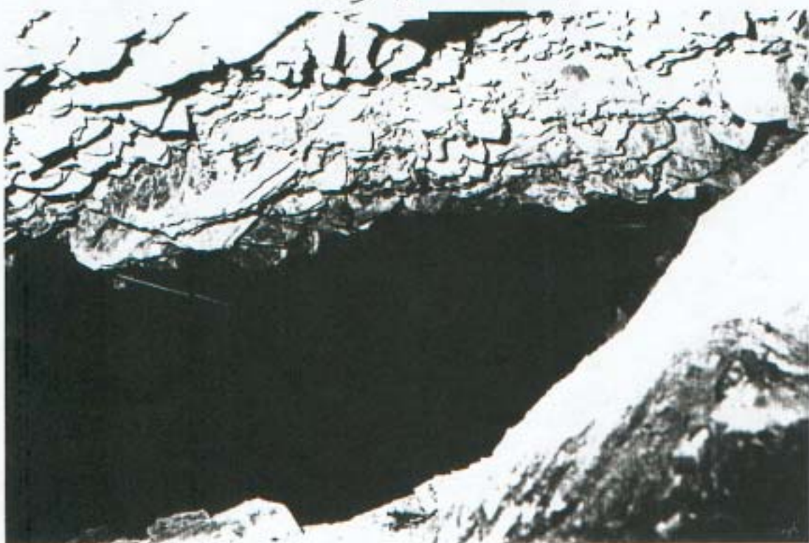
View Looking into Cavity Showing Extent of Roof Fall. Location 7 Face
