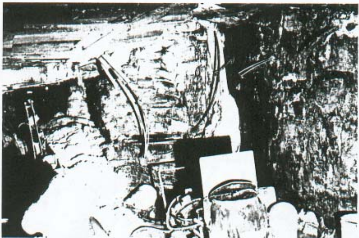
R.H. TOP CORNER SHOWS INJECTION TUBES INTO COAL FACE AND ROOF TO BIND STRATA IN ADVANCE OF ROOF CAVITY.
