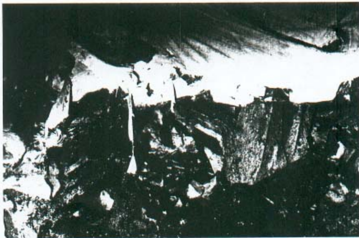
Fallen Roof Stone Protruding Through Polyurethane Block
