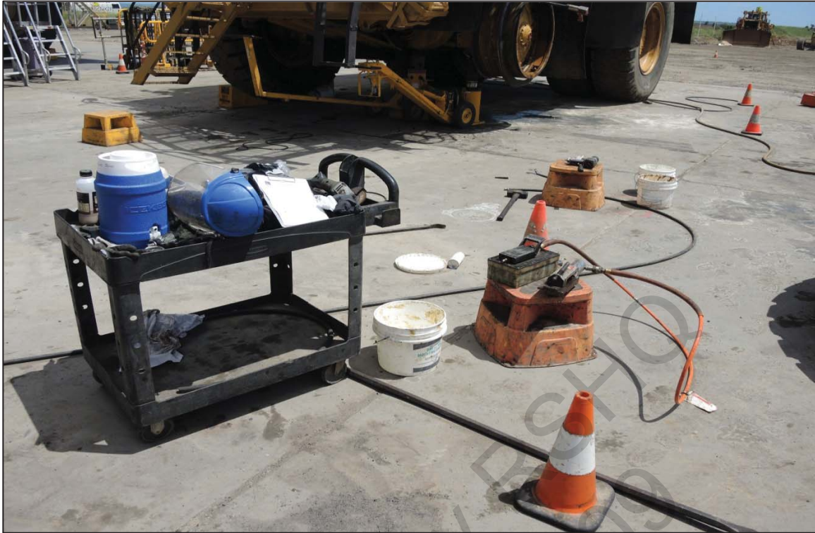
Figure 5: Bead Seat Breaker on the Orange Step (DNRM photos taken at the incident scene).
