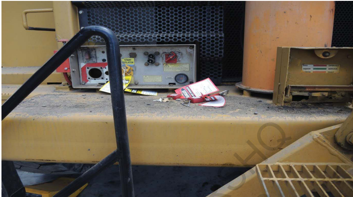
Figure 4 sch4p4( 6) Personal information danger tags and personal locks not applied to the isolation point of the truck (DNRM photo taken at the incident scene).
