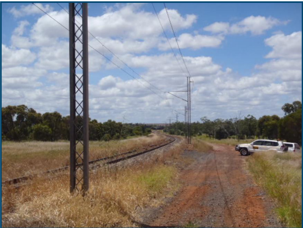
Picture 6: View east from Occupational Crossing 5805
