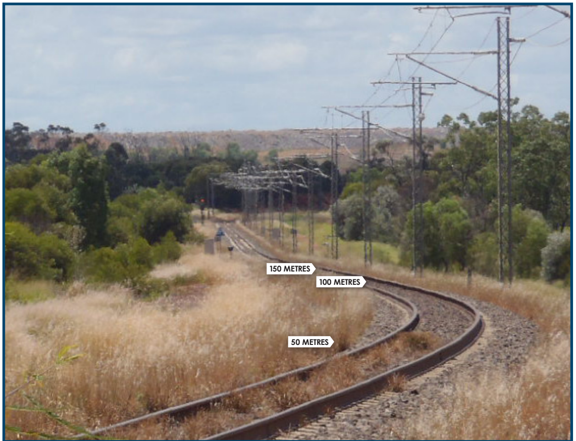
Picture 7: Curvature of track (showing distances from 5805)
