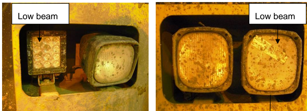
Figure 24. RHS (below left) and LHS (below right) front lighting (low beam and high beam) of truck. Photographs taken by investigators on 5 December 2013.
