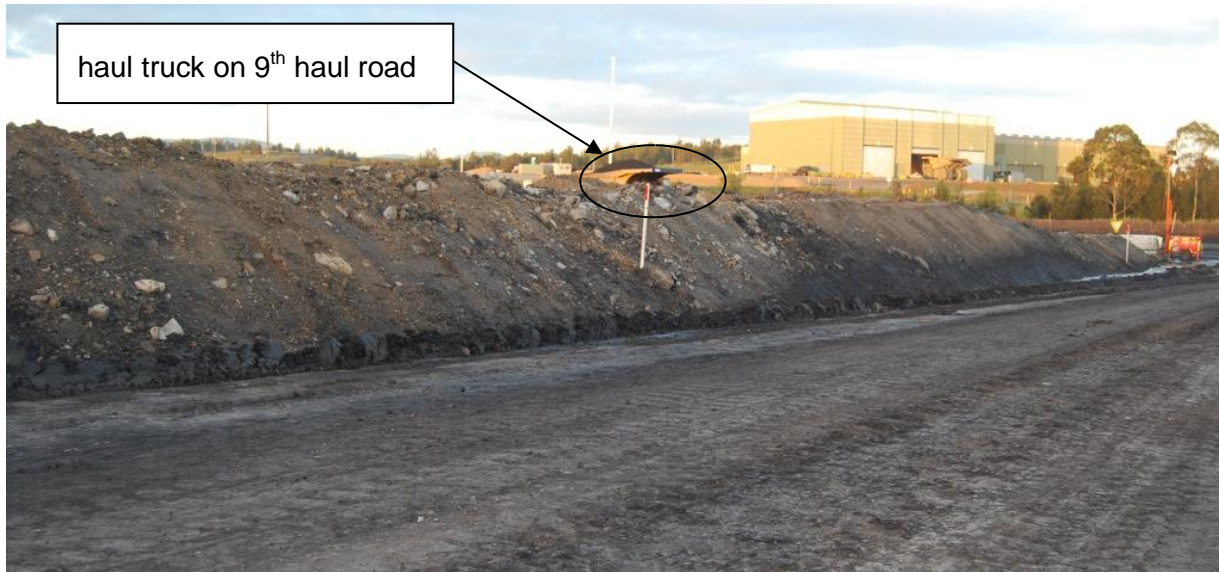
Figure 13. Photograph of windrow on 8 th ramp taken by investigators at the mine on 1 December 2013.
