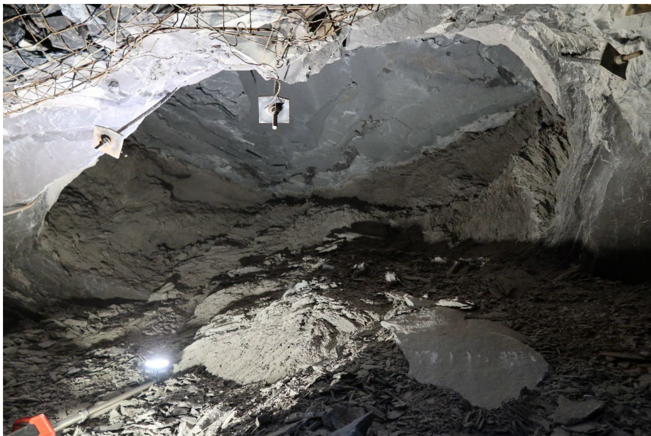
Figure 3: The void above the coalface in Razorback Mains B heading 11-12 cut-through
