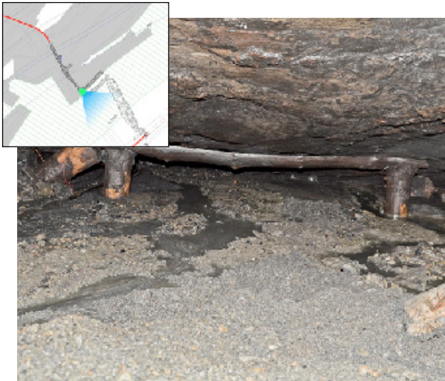
Figure 12 Silt and debris at the bottom of the Top Road
