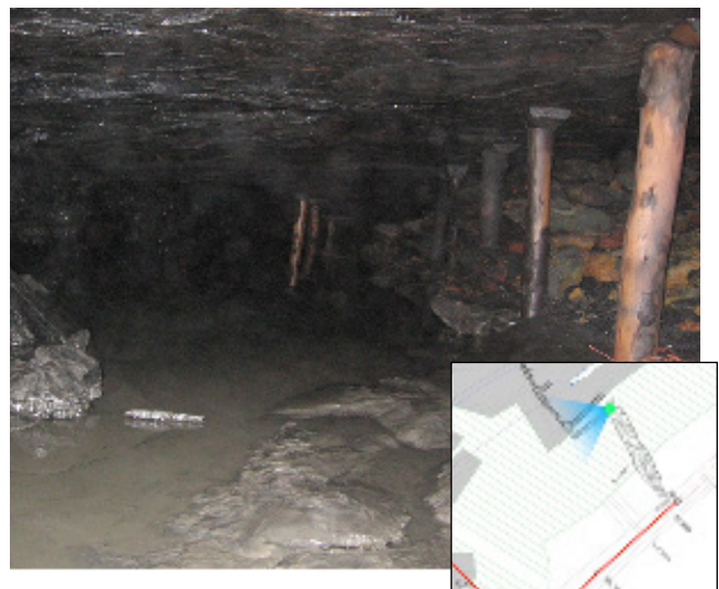
Figure 18 Looking from the breach along the bottom edge of the Old Central Workings back towards the bottom of the Top Road. Wooden props and stone packs are intact. Only some of the silt seems to have been washed away within a few metres of the breach
