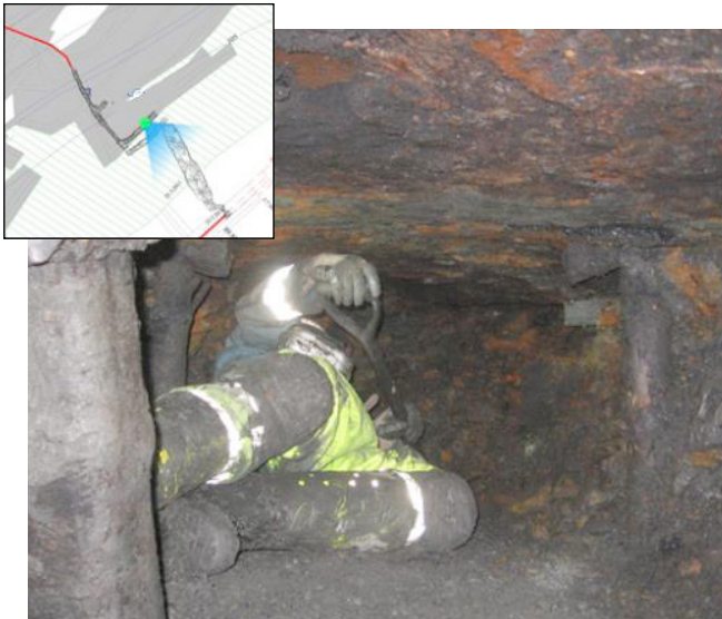
Figure 16 Mines rescue workers tunnel through the stone pack in the Old Central Workings to gain access to the breach from the opposite side to the inrush stall
