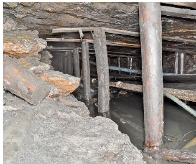
Figure 3 The entrance to the H1 roadway from the Main Drift, taken after the inrush; some water and silt can be seen beneath the conveyor towards the bottom right
