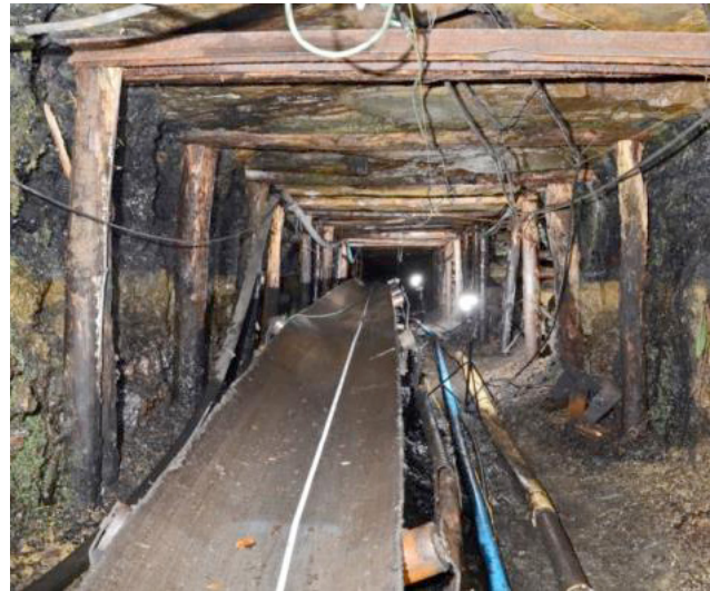
Figure 2 View looking down the Main Drift – the main way into the mine
