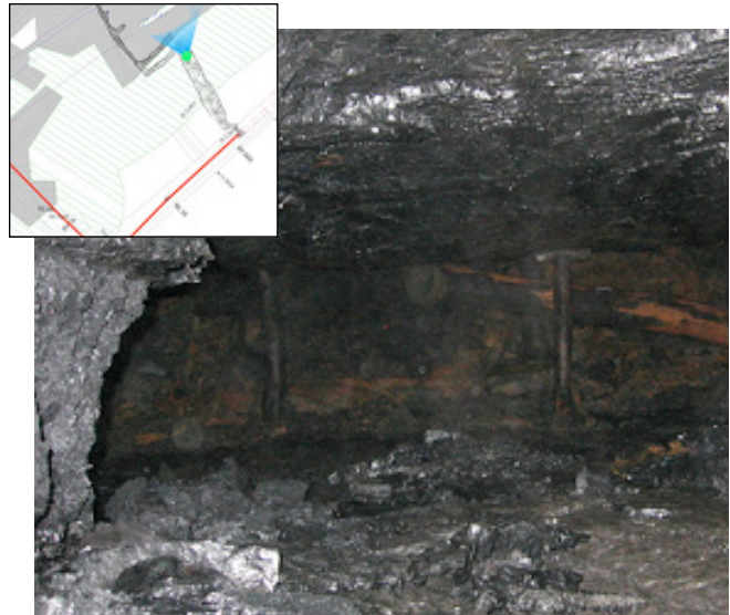
Figure 15 The breach at the top of the inrush stall into the Old Central Workings. The props set and the stone packs built when coal was extracted from there in the 1980s can just be seen through the breach
