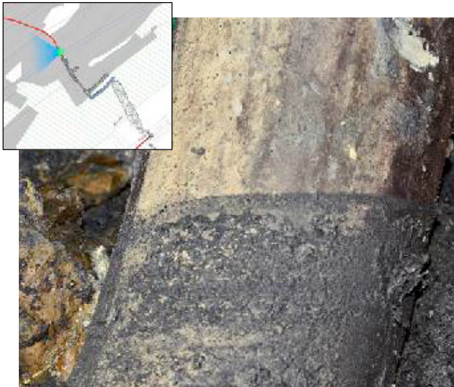
Figure 10 Tide mark on wooden prop in the Top Road approximately 214 m from the mine entrance. The level of the mark is at 109 m above sea level
