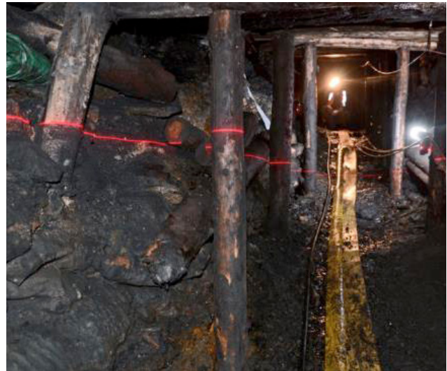
Figure 11 A laser level picks out the tide marks in the Top Road within the Old Central Workings
