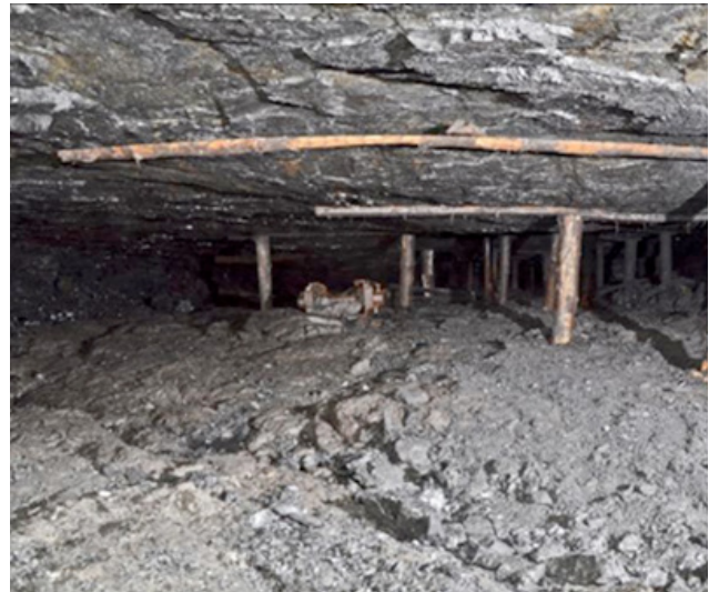
Figure 17 View into the inrush stall from the position of the breach
