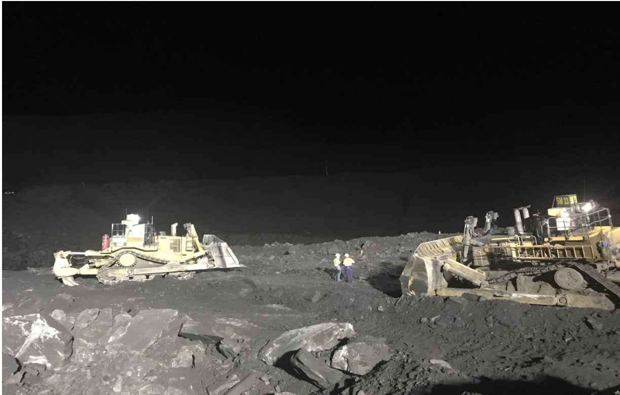
Position of dozers during illumination testing.
