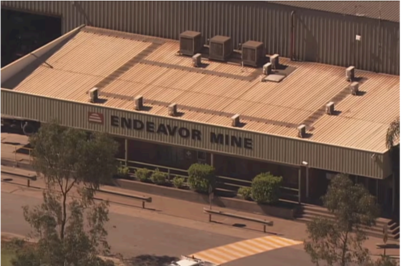
Emergency service crews were called to the mine on Endeavor Mine Road at Cobar. (ABC News)
